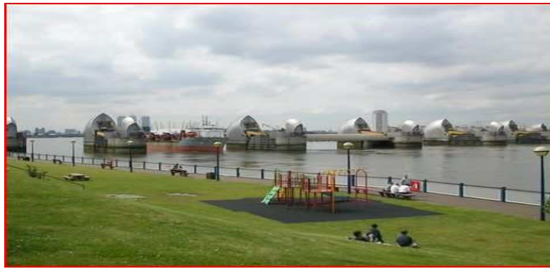
Thames Tidal Barrier
